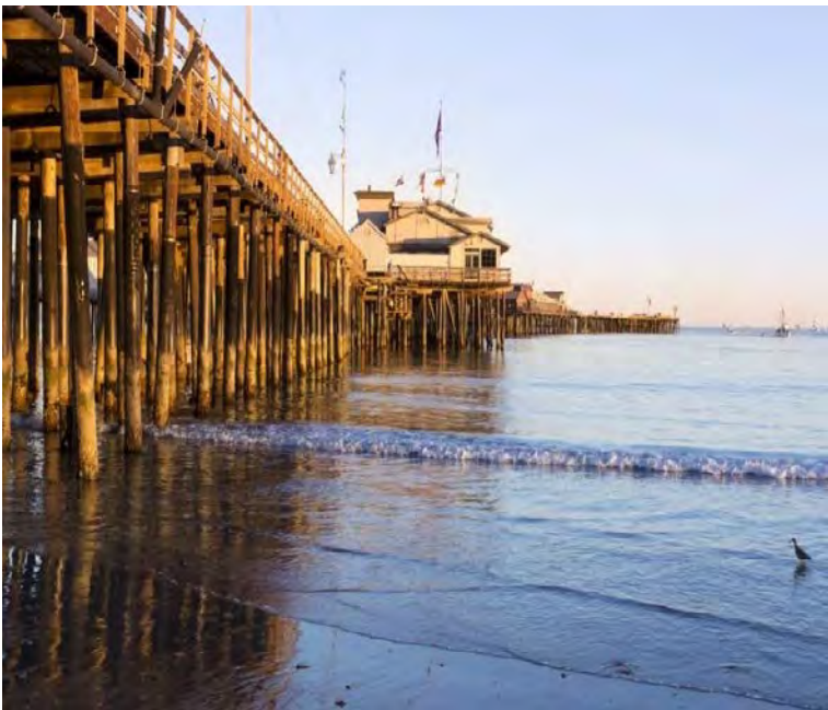
Santa Barbara Stearns Wharf
